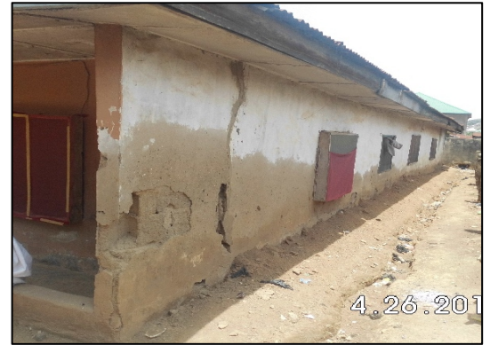
Figure 1: High vulnerability class. Buildings with poor building material, building condition and building quality. NB: Please use these buildings only for ASSESSMENT SHEET 1 - Table 1
