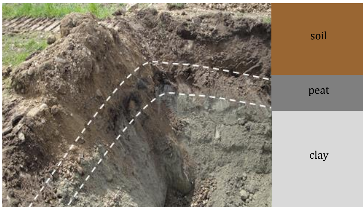
Fig. 25: Collection of peat samples during canalization works in June 2014 (Photo: Heinz Surbeck). Above the peat horizon there is approximately 0.5 m soil and below there is a clay layer.
