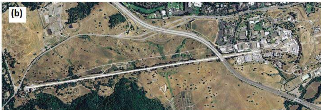
Fig. 1.110: a) Two installed side by side linacs with 15kW and 10MeV incident electron beam energy in a medical products sterilization facility. b) a 3.2-kilometer linear accelerator installed at the Stanford Linear Accelerator Center that enables it to accelerate electrons to 50 GeV [HH12, SLAC]
