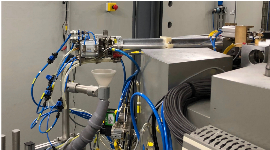
Figure 2.4: The STS installed on the out-port 7 of the Bern medical cyclotron.
