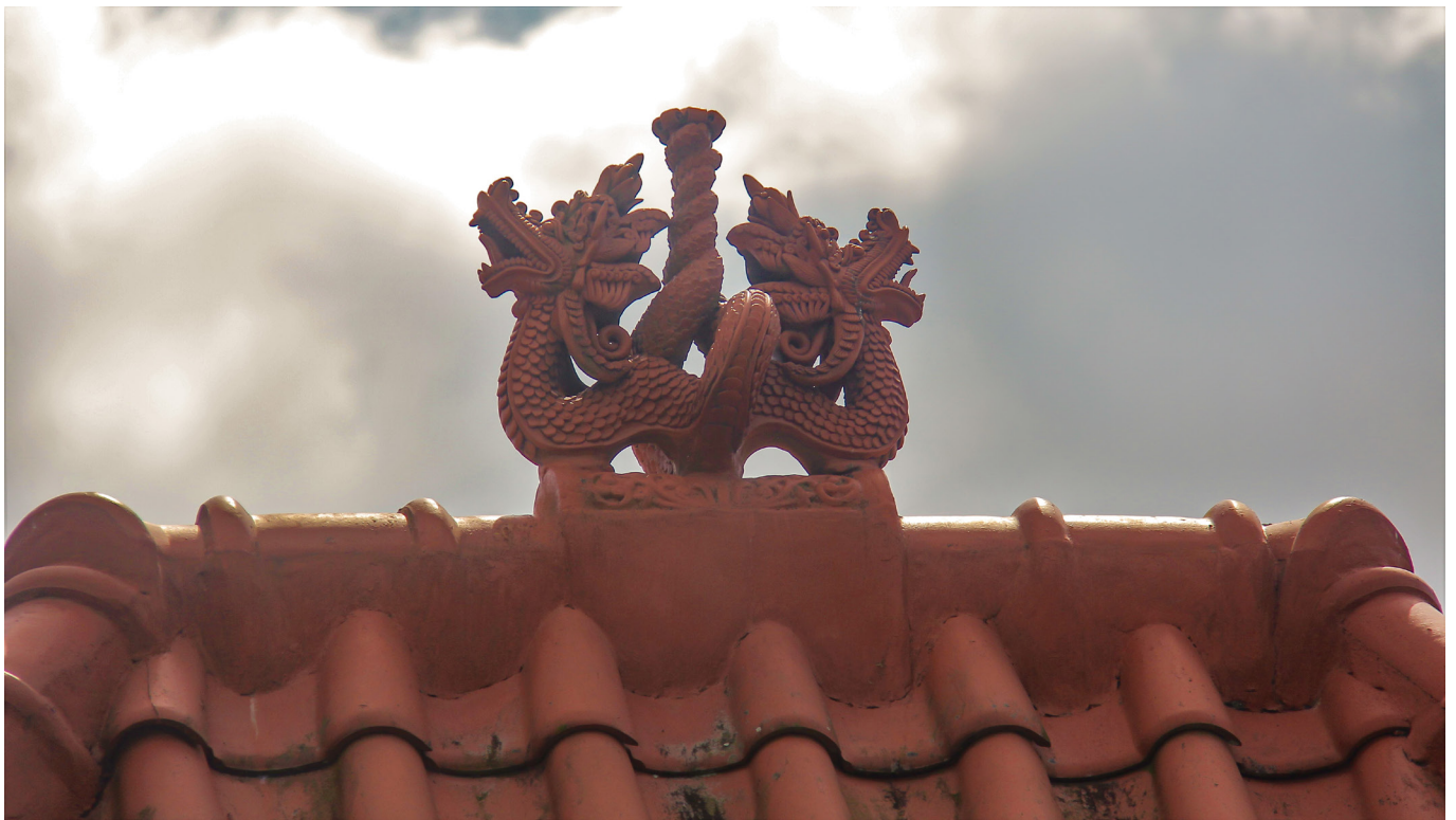
Figure C7 Symmetric wuwungan (roof top decoration) with a two naga (snake). made with the teknik tempel (glueing technique), by potters from Kasongan. Image by Wahyu Priyono.
