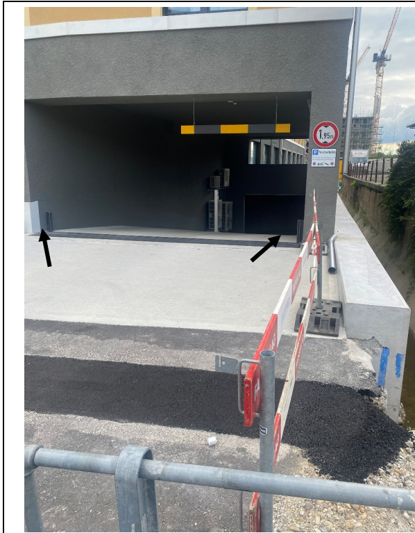
Figure 4-3. Example of a newly-built building in the medium hazard zone and two implemented PLFRA measures at the entrance of an underground parking garage (elevated entrance and devices for temporary embankments (black arrow)).
