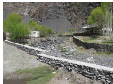
Figure 97: Dam construction to protect the village (Source: Zimmermann, 2013)
