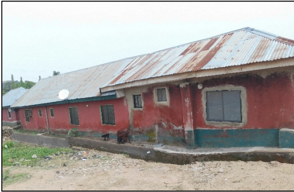
Figure 1: High vulnerability class. Buildings with poor building material, building condition and building quality. NB: Please use these buildings only for ASSESSMENT SHEET 1 - Table 1
