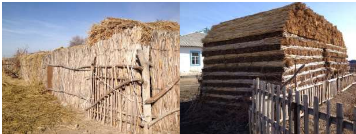
Figure 5.2. Reed bundles are used for construction in the Syr Darya Delta
